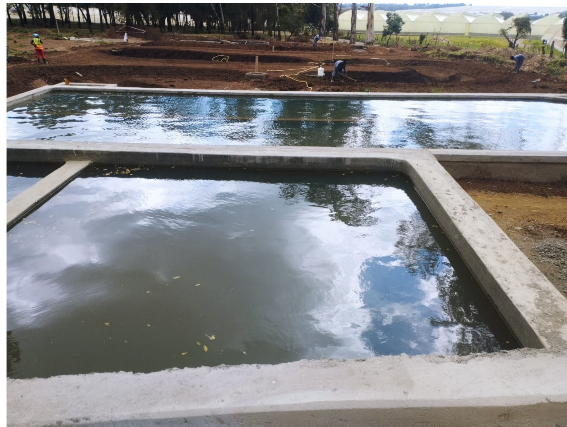
Construction of a waste water treatment system (wetland) in progress
